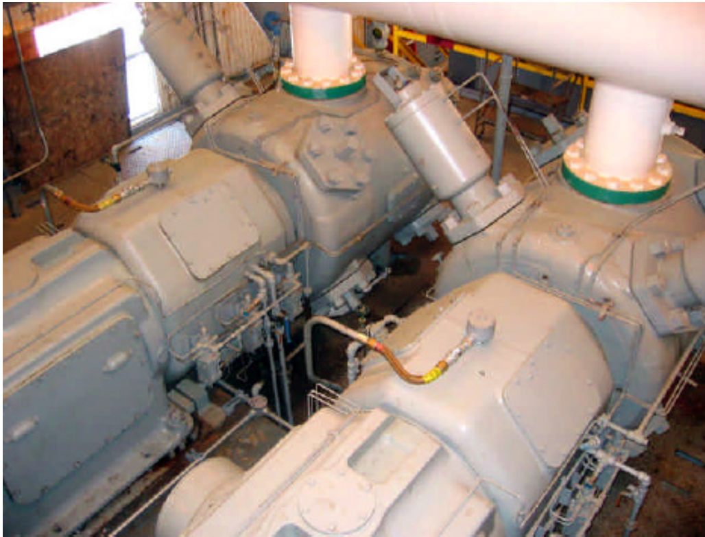
IT6810 Impact Transmitters Mounted on the Crosshead
