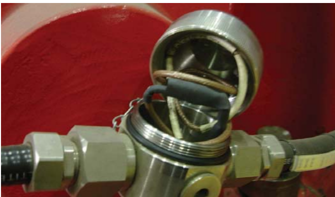
Conventional connection ends with stuffed-in cables.
