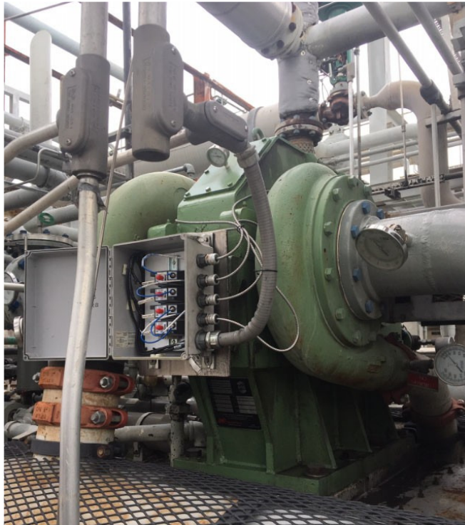
Figure 2. One typical application of a Centrifugal Air Compressor
